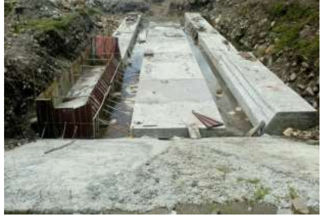
M15 concrete works at the base of desilting basin
