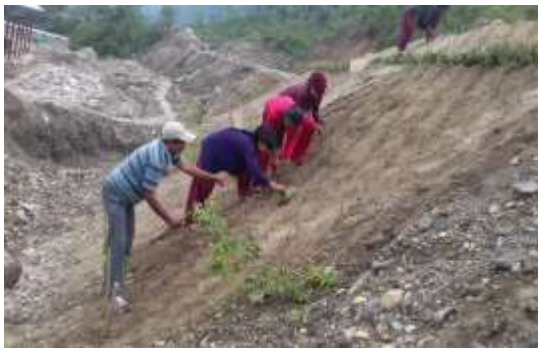
Bio-engineering Works along WCP alignment
