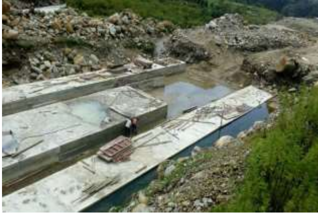
M15 concrete works at the base of desilting basin
