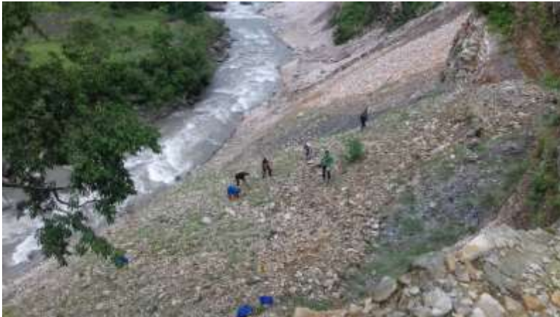
Bio-engineering Works Along WCP alignment
