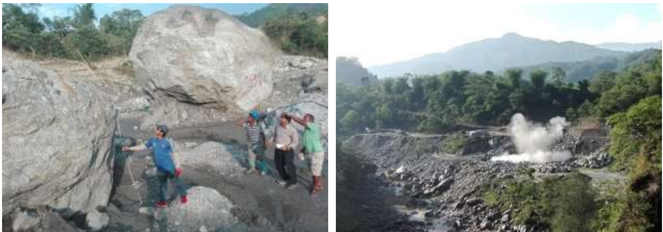
Big boulders at powerhouse and blasting in progress.
