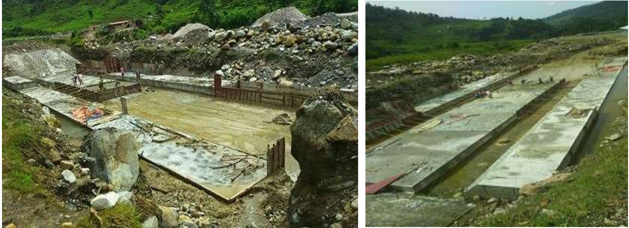
M15 concrete works at the base of desilting basin
