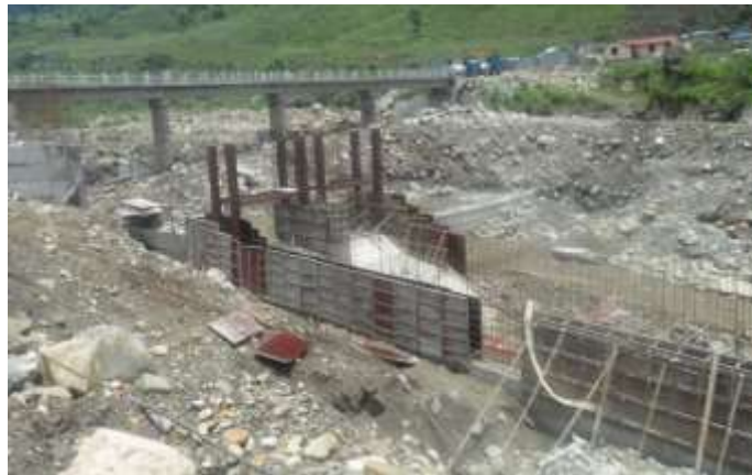
Construction work of Undersluice
