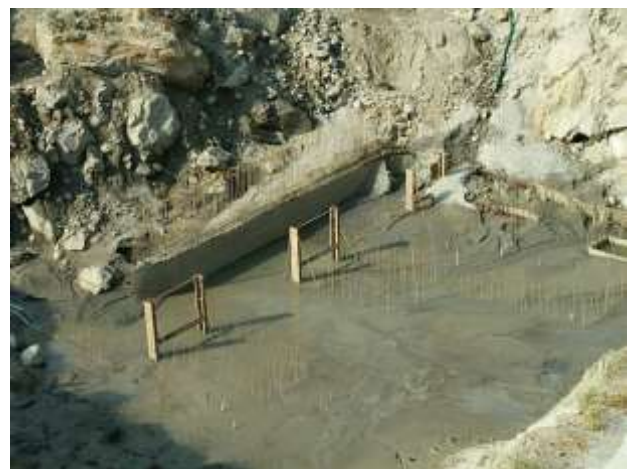
Dewatering and debris cleaning at Powerhouse
