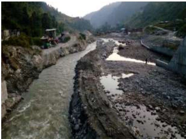
River Diversion from Left Bank
