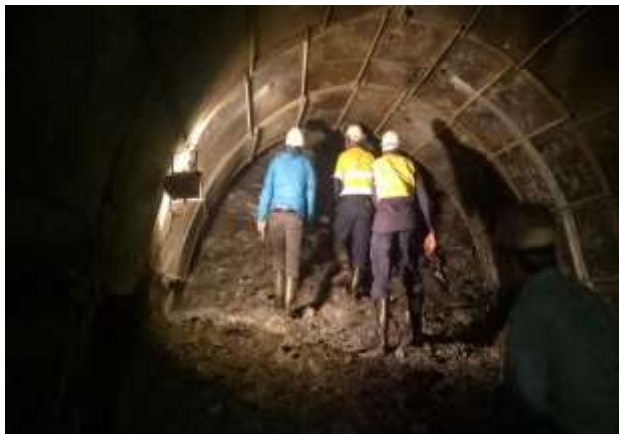
Inspection of inlet Tunnel face after Heading Blast Outlet Tunnel Face; installing initial supports
