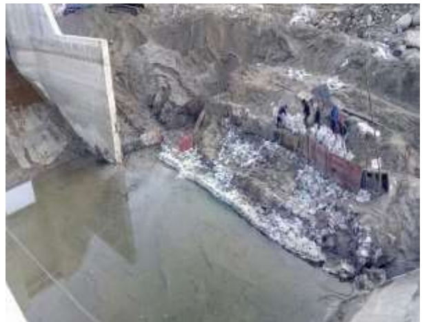
Cleaning of Debris at downstream of weir
