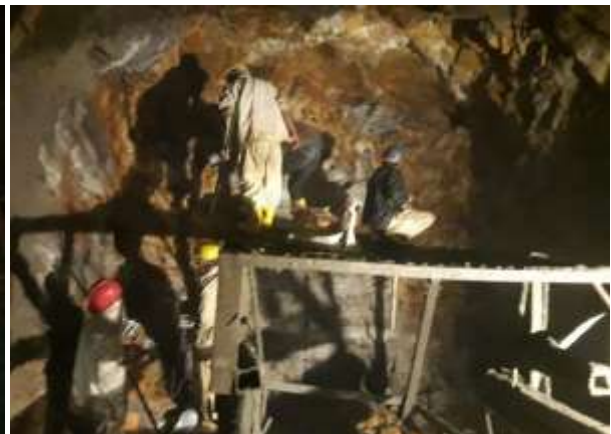
Inspection of inlet Tunnel face after Heading Blast Outlet Tunnel Face; installing initial supports
