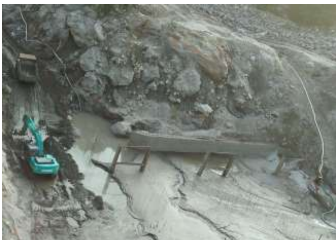
Dewatering and debris cleaning at Powerhouse
