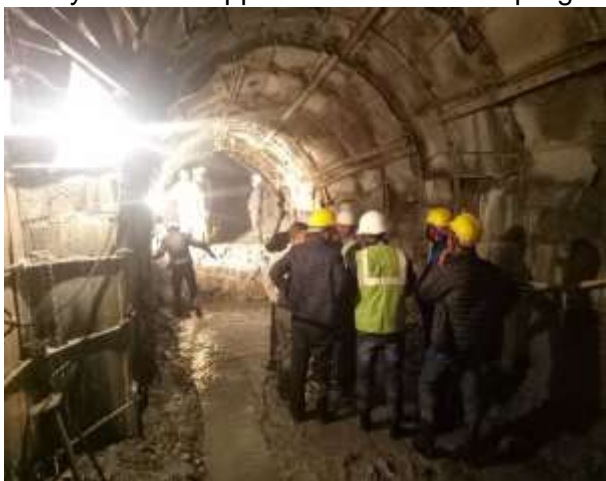
Inlet Tunnel face
