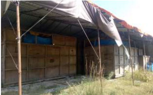
Electro-Mechanical Equipment Stored at army yard
