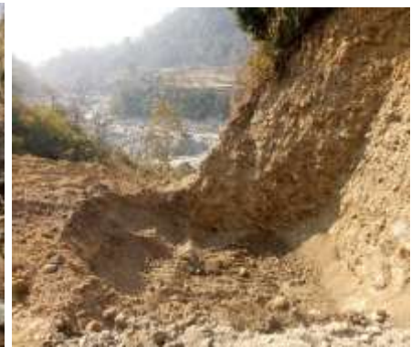
Penstock Pipe Alignment and excavation of Anchor Block AB-06
