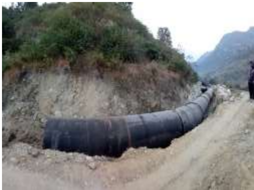
WCP Alignment Excavation and installation of pipes
