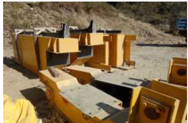
EOT Crane Parts Delivered at Project Site
