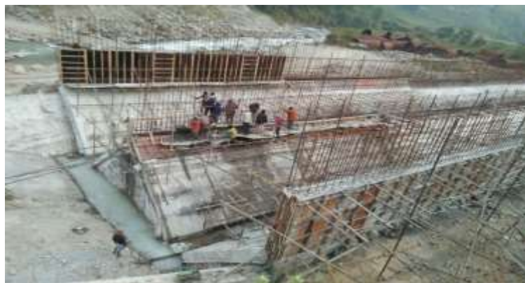
Desilting Basin Construction
