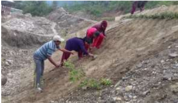
Bio-engineering Works Along WCP alignment
