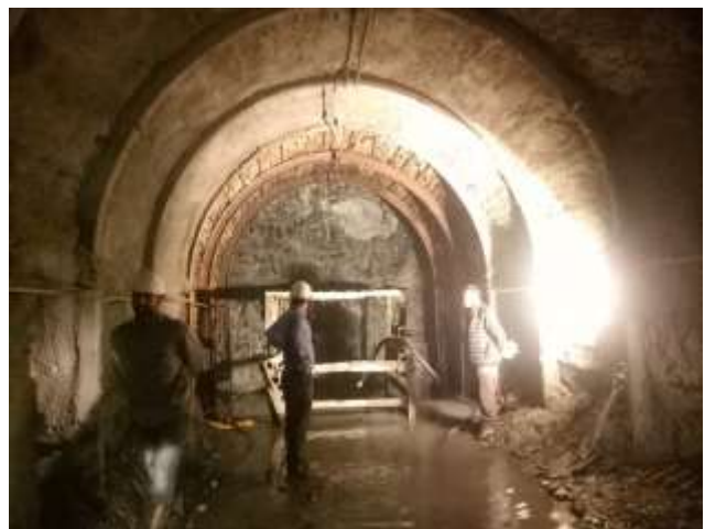
Outlet Tunnel Face
