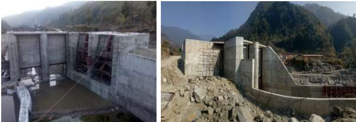
Intake and Undersluice Structures
