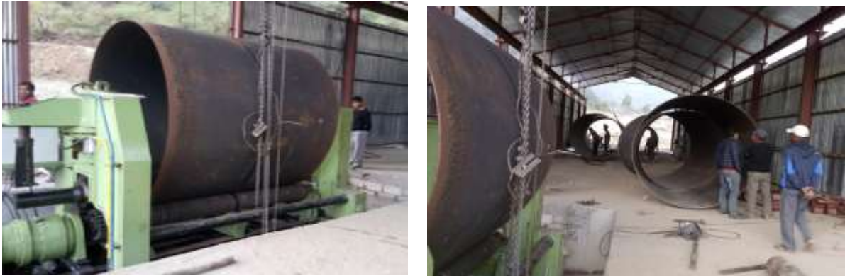
HM Workshop and Pipe Rolling /welding
