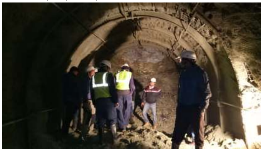
Tunnel Excavation from Outlet. @CH 187 m
