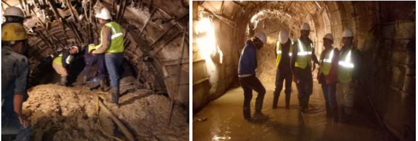
Rectification and further advancing from Inlet
