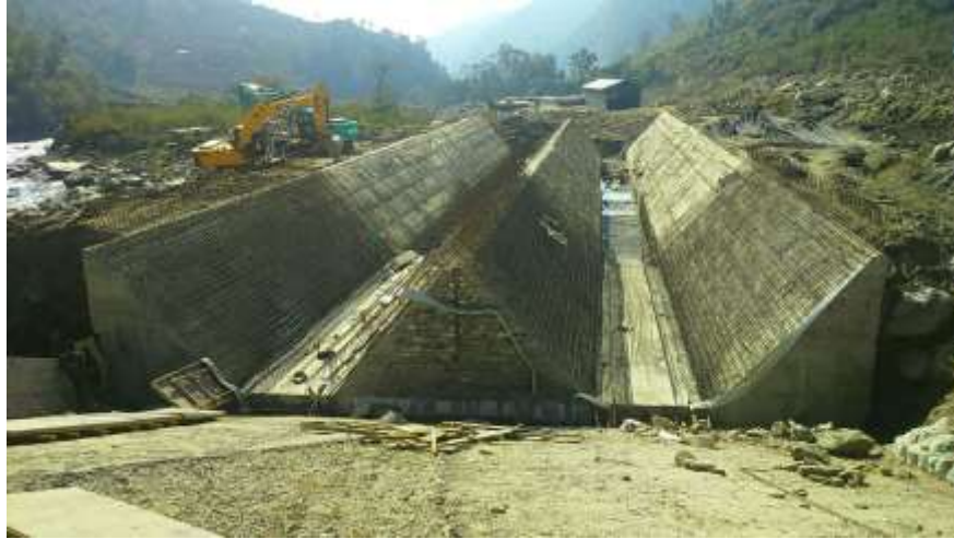
Construction activities at desilting Basin Structure
