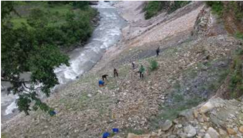
Bio-engineering Works Along WCP alignment
